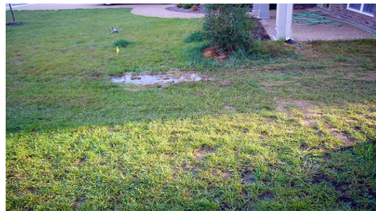
Figure 2 – Negative Drainage
